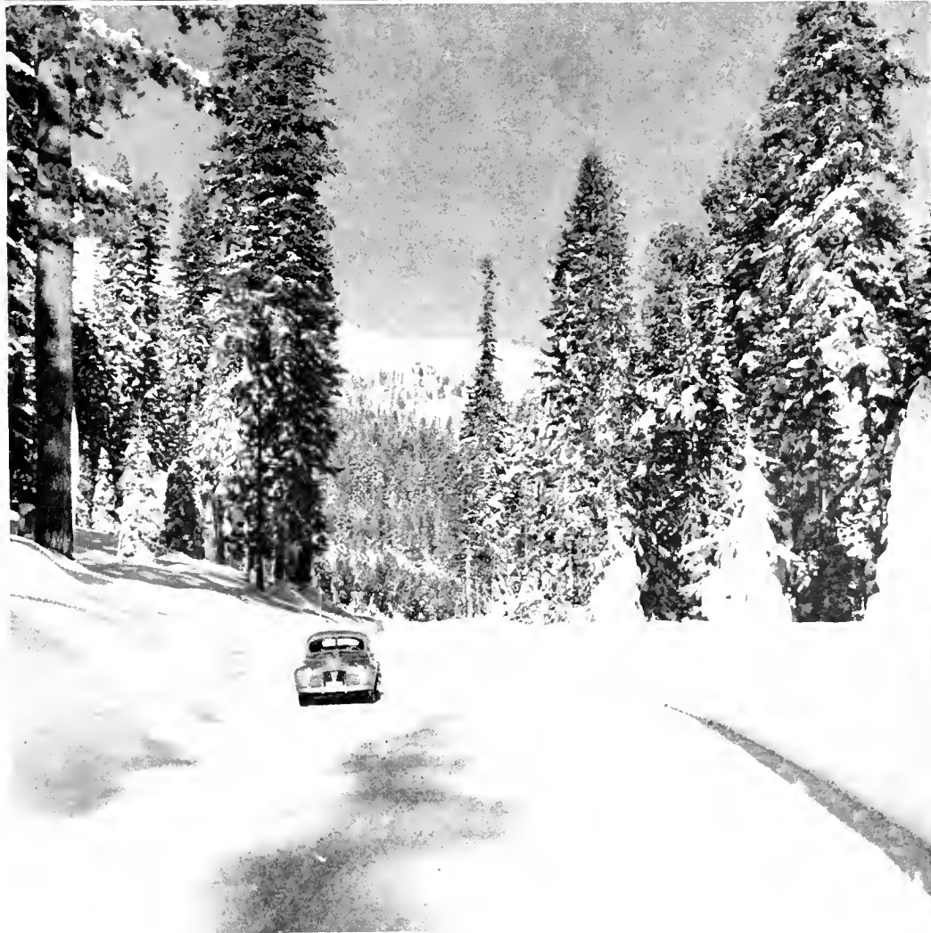
Upper—New maintenance station of Division of Highways on Echo Summit Lower—View on U. S. 50 west of summit
